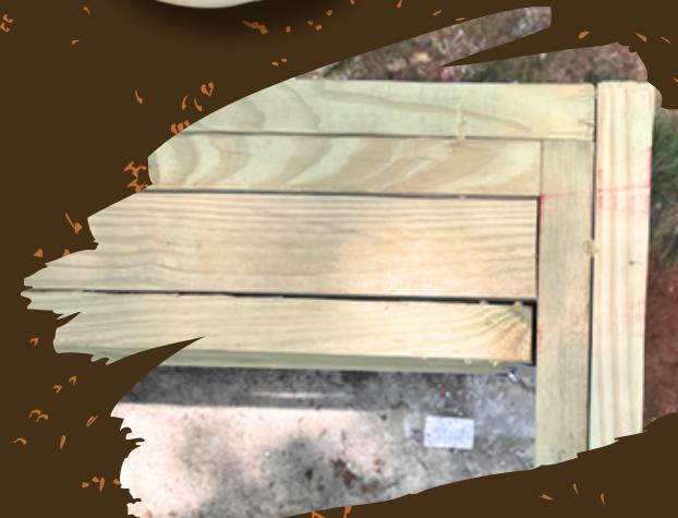
Heavy, Thick, or Flat Blocking suffocates the boards from below and causes Cupping
