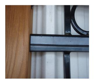
**Adjustable Connectors** are available in both the hidden and collar styles. The vertical adjustable connectors are used for stair rails and the horizontal adjustable connectors are used for railings that meet the post in other than a 90 degree angle.
